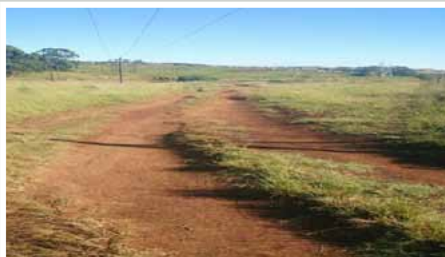
Ntendeka New Gravel Road before Construction
