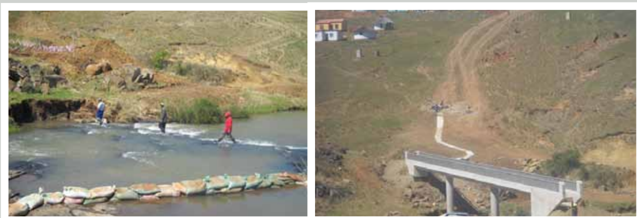
3374 Weza River Pedestrian Bridge Site before and after Construction
