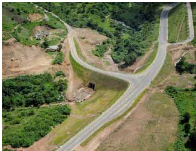
P100 and P102 intersection – after construction
