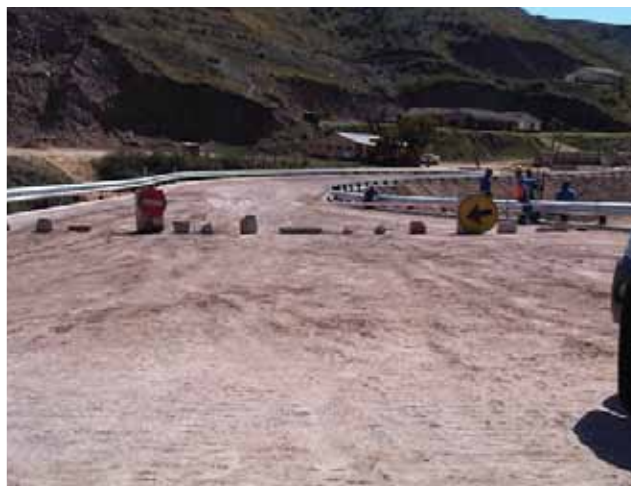
P100 and P102 intersection - during construction
