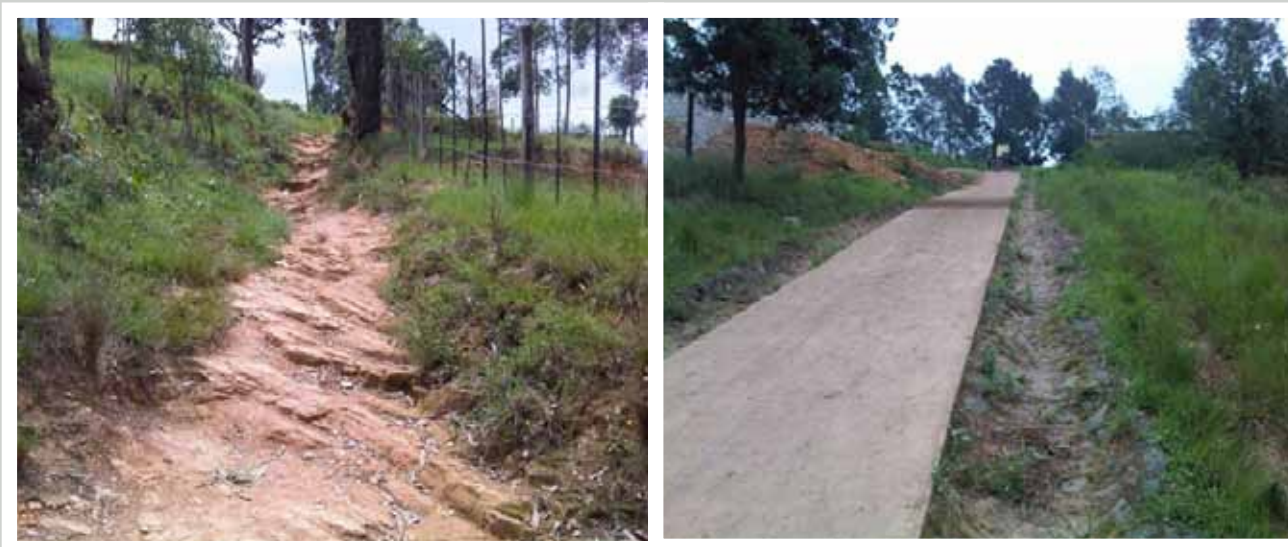
Ndlela Access Road before and after construction
